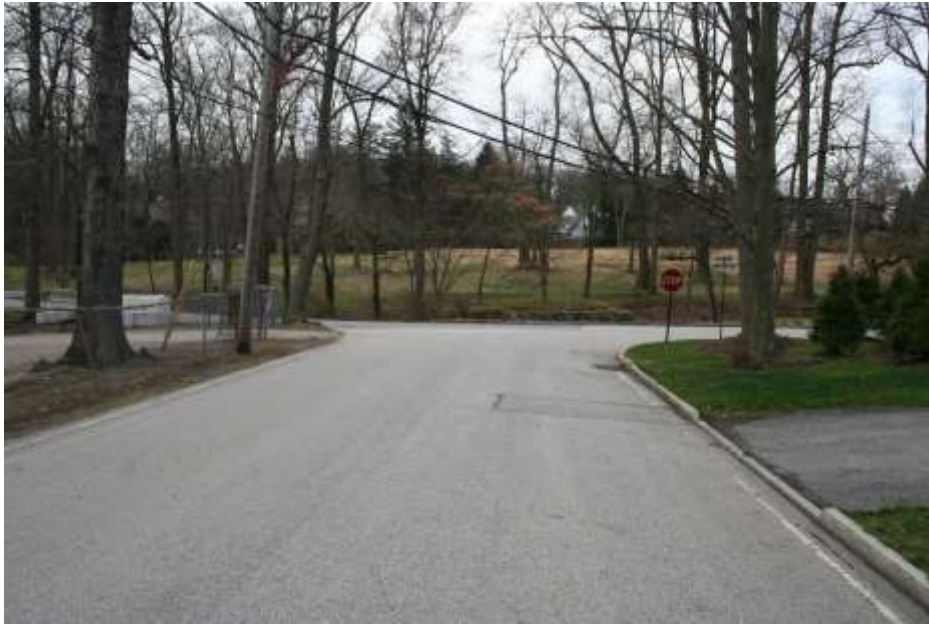
Photo # 1 - Description: Southbound Paul Road approaching Walnut/Chamounix (~ 50')
