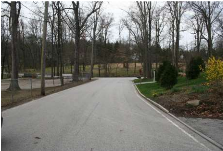
Photo # 2 - Description: Southbound Paul Road approaching Walnut/Chamounix (~150')
