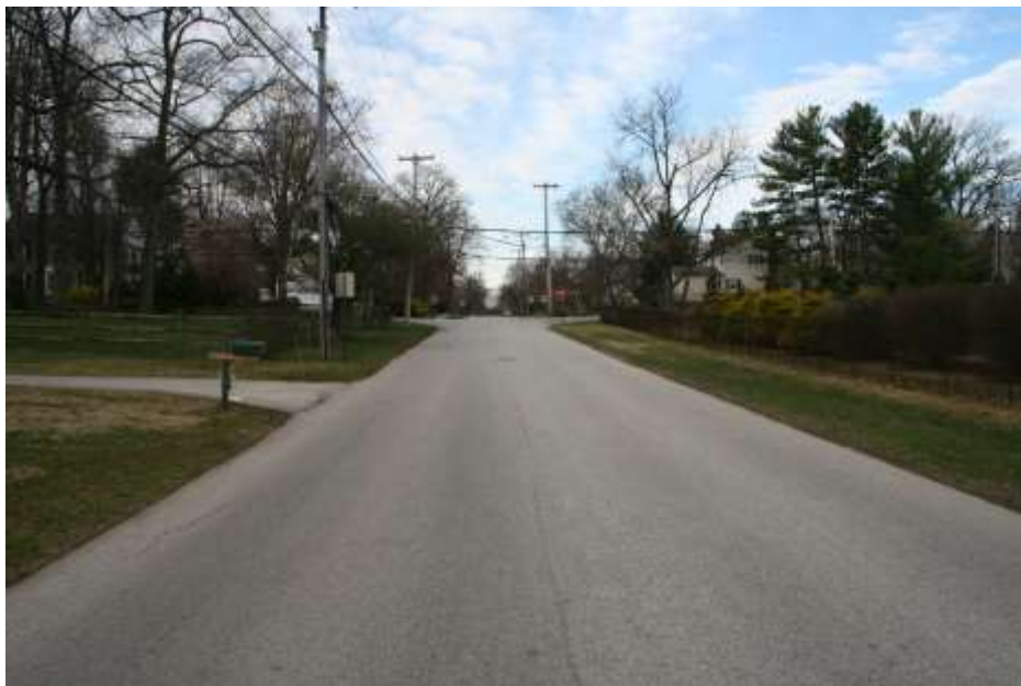
Photo # 6 - Description: Westbound Walnut Avenue approaching Radnor Street Road (~200')
