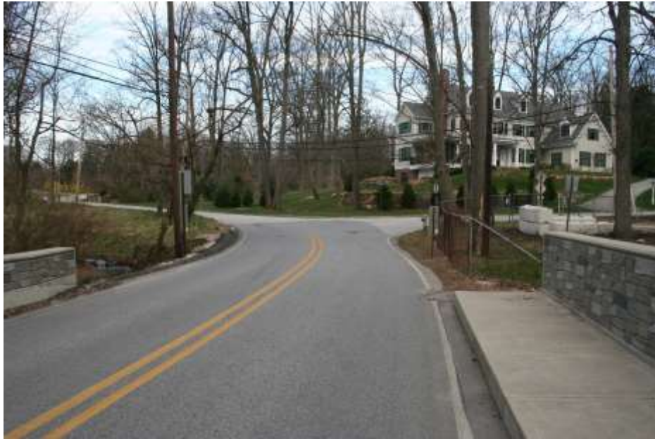
Photo # 3 - Description: Westbound Chamounix approaching Paul Road (~50')
