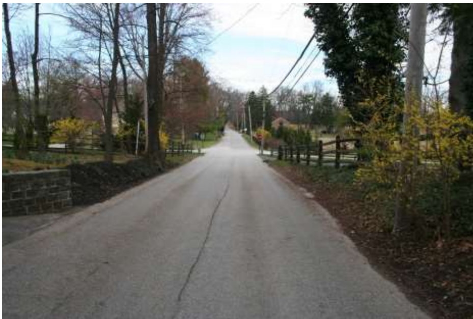
Photo # 2 - Description: Northbound Radnor Street Road approaching Walnut Avenue (~150')
