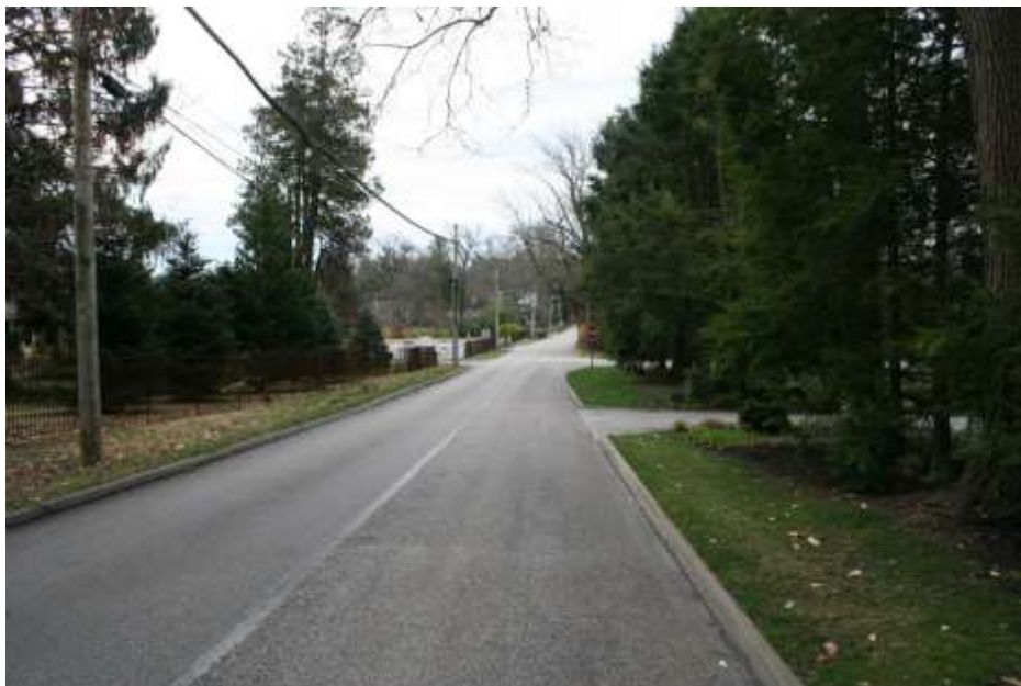
Photo # 4 - Description: Southbound Radnor Street Road approaching Beechtree Lane (~200')
