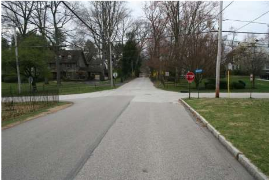
Photo # 3 - Description: Southbound Radnor Street Road approaching Walnut Avenue (~50')
