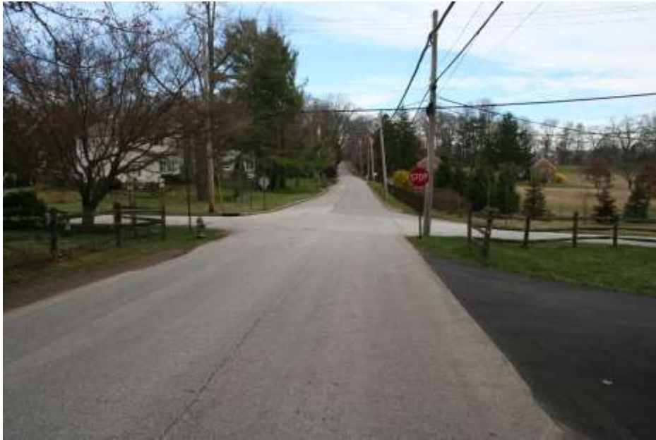
Photo # 1 - Description: Northbound Radnor Street Road approaching Walnut Avenue (~ 50')
