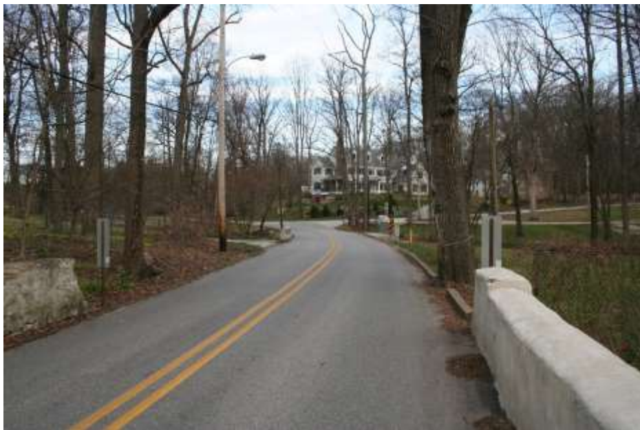
Photo # 4 - Description: Westbound Chamounix approaching Paul Road (~200')
