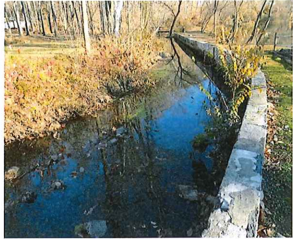
Downstream Retaining Wall – Looking Downstream
