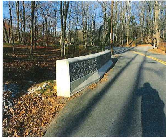
Bridge Barrier on a Newly Constructed Bridge along Chamounix Road over Branch of Gulph Creek
