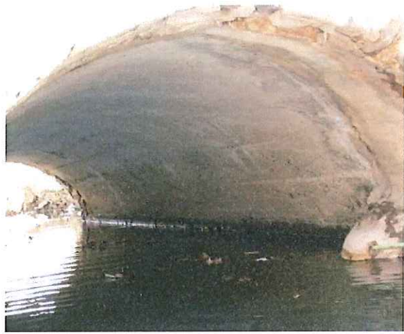
View of Concrete Arch North Barrel
