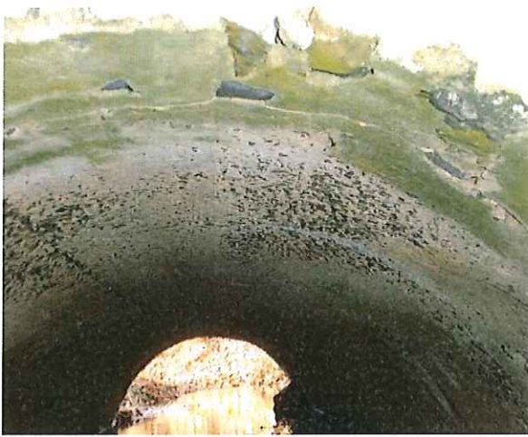
View of Concrete Arch South Barrel
