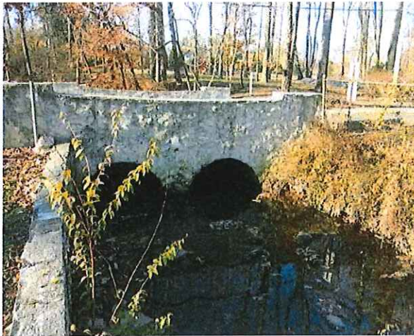
Downstream Retaining Wall – Looking Upstream
