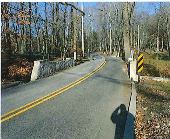
General View of Culvert – Looking North
