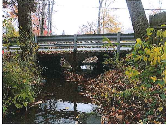
North Grouted Masonry Headwall
