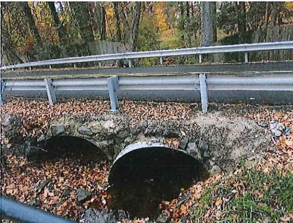
Guiderail Posts at South Fascia
