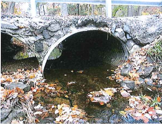
South Grouted Masonry Headwall
