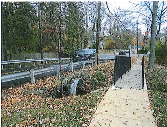
General View of Culvert and Pedestrian Bridge
