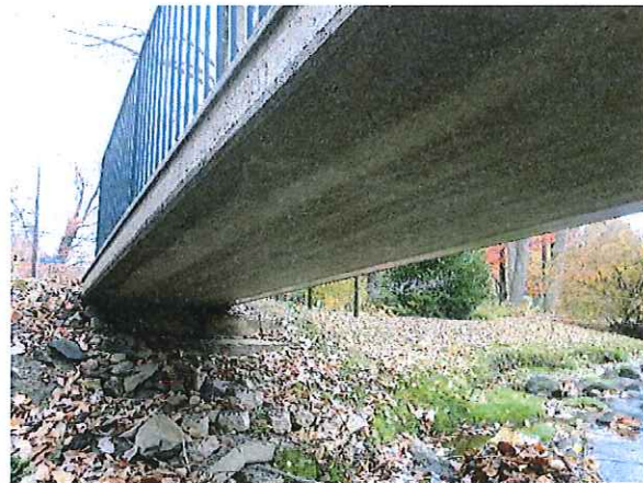
Underdeck View of Pedestrian Bridge
