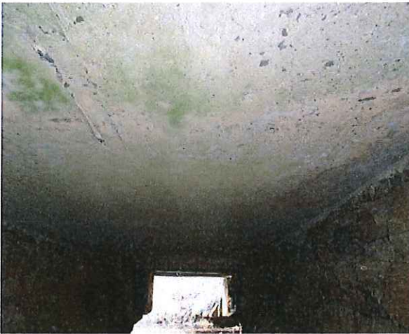
View of Original Concrete Slab Superstructure (underside)
