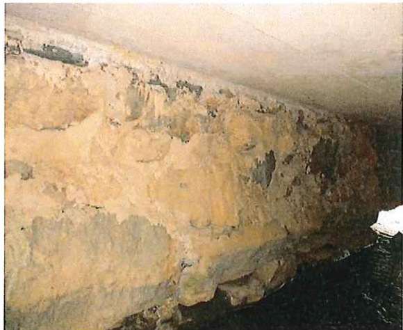
View of Original South Stone Masonry Abutment
