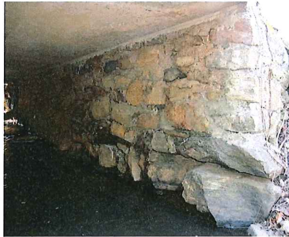
View of Original North Stone Masonry Abutment
