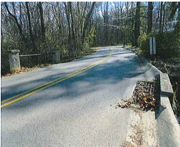
General View of Culvert – Looking South. Note Inlet Structure in West Shoulder
