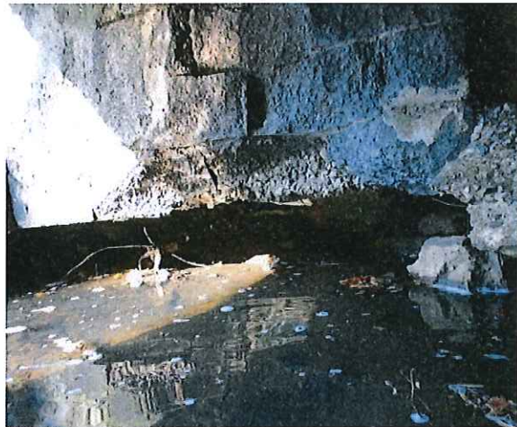
North Abutment of Inlet Structure – Looking Southwest
