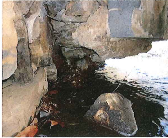
South Abutment of Inlet Structure – Looking Southwest
