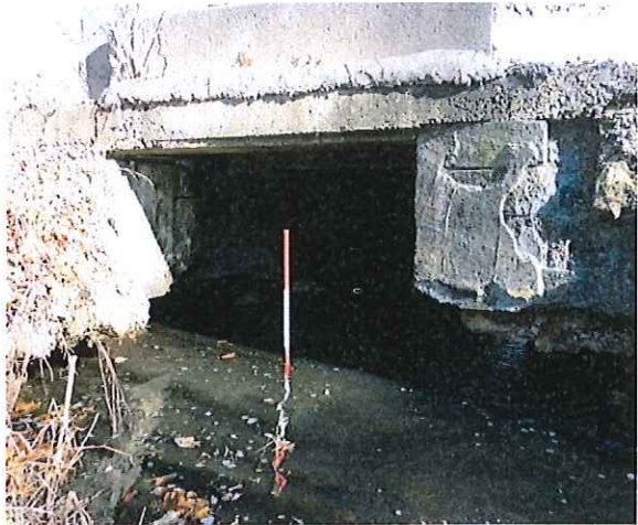
West Fascia - Inlet Structure
