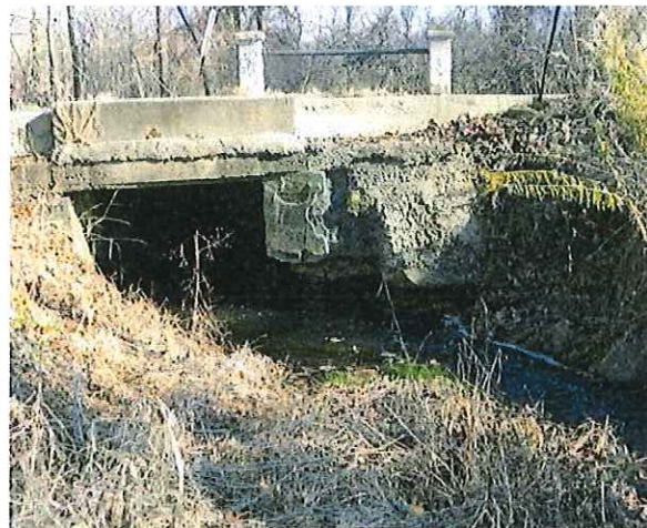
Upstream Elevation. Note Stream Flow Entering the Culvert with a Sharp Skew and Skew of the Culvert
