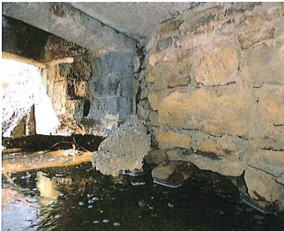
North Abutment of Inlet Structure – Looking Northwest
