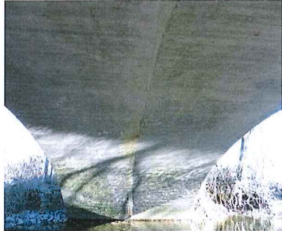
Concrete Arch Barrel – Looking at East Abutment
