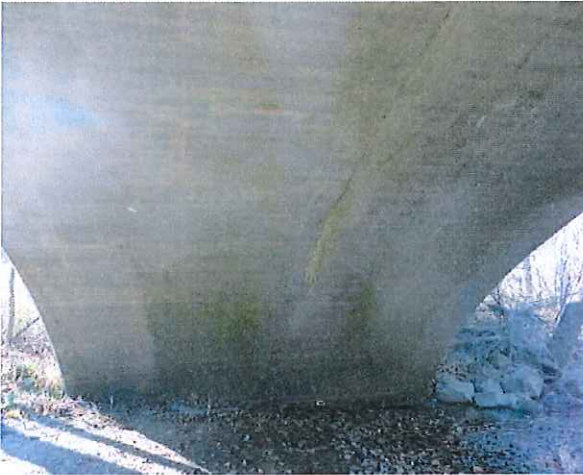
Concrete Arch Barrel – Looking at West Abutment
