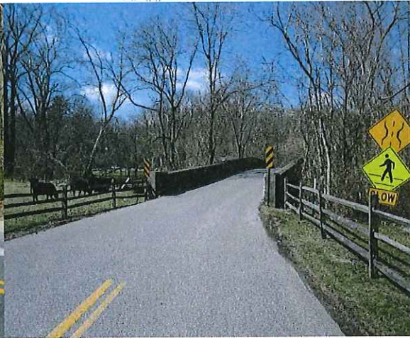
East Approach, Note Sign of Pedestrian Crossing
