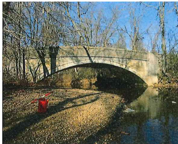
Downstream (South) Elevation
