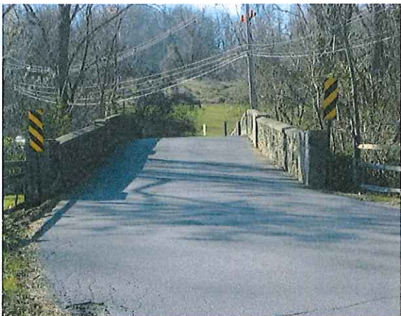
General View of Arch Bridge – Looking East
