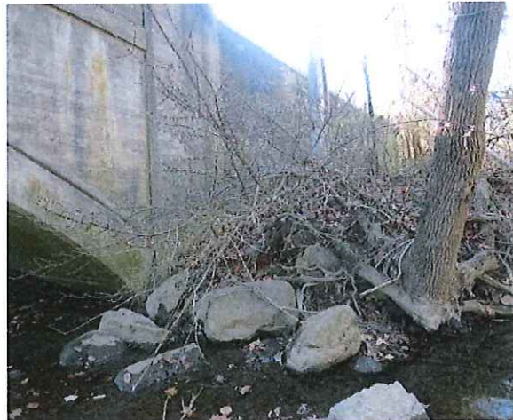
Upstream Right Bank at West Abutment
