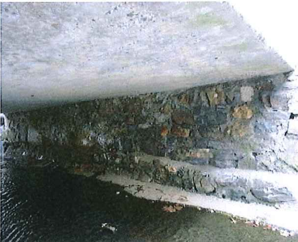
Typical Masonry Abutment
