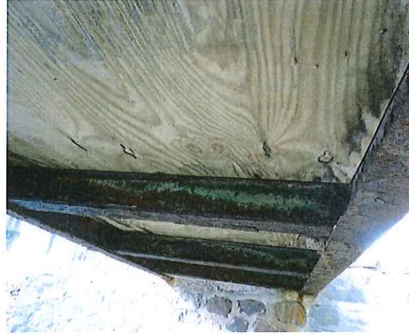
South Pedestrian Bridge Underdeck View
