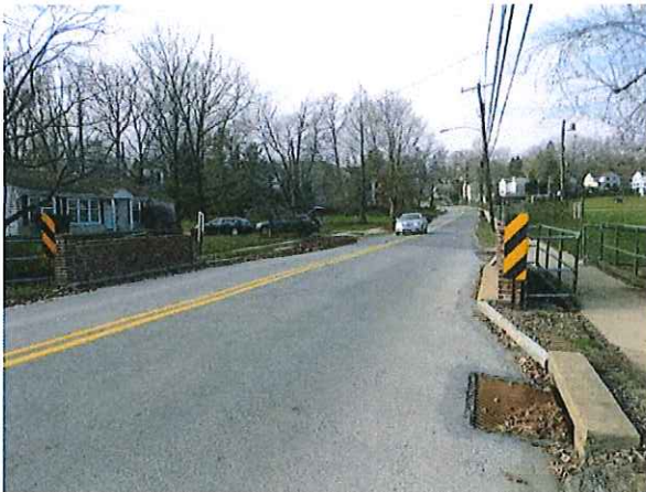
General View of Roadway and Pedestrian Bridges Looking West
