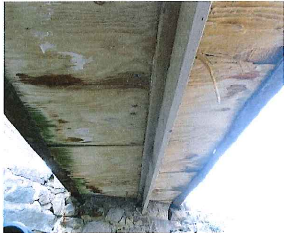
North Pedestrian Bridge Underdeck View
