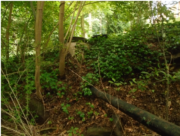
Exposed 6" sewer and manhole on west embankment
