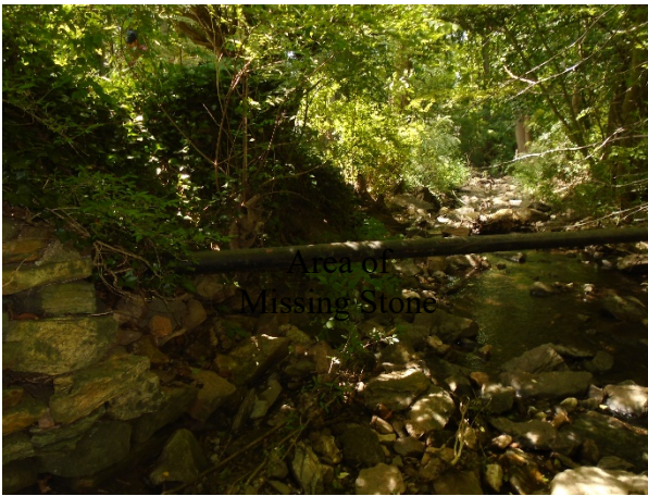
6" exposed sewer lateral downstream
