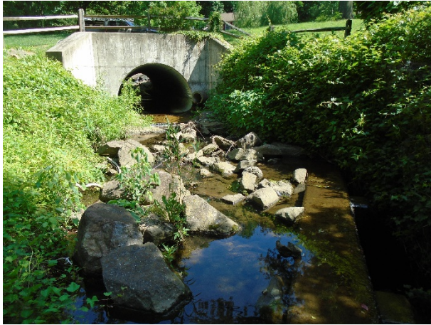
General View of Pipe Culvert from downstream
