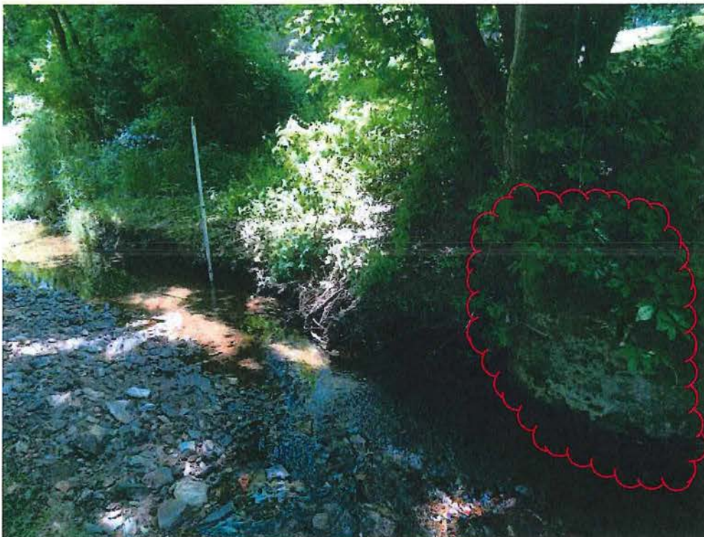
Photo 4. Undercut and eroded banks downstream of manhole.
