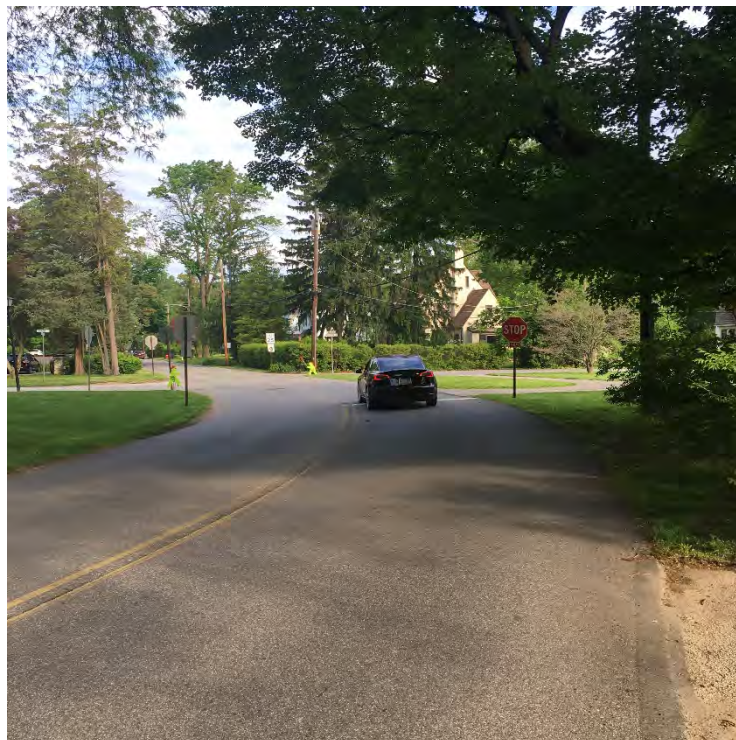
Photo # 2 - Description: Westbound Strafford Road
