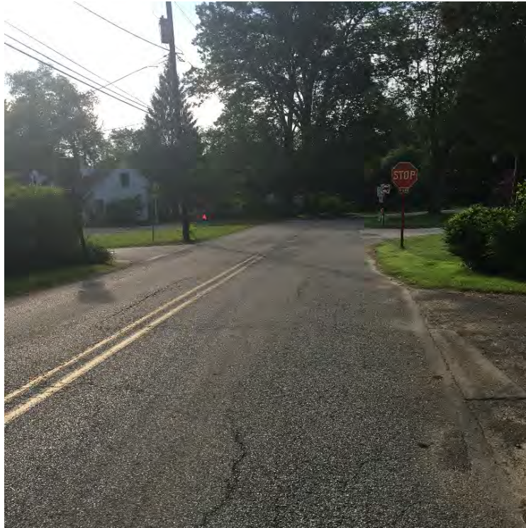
Photo # 1 - Description: Eastbound Strafford Road
