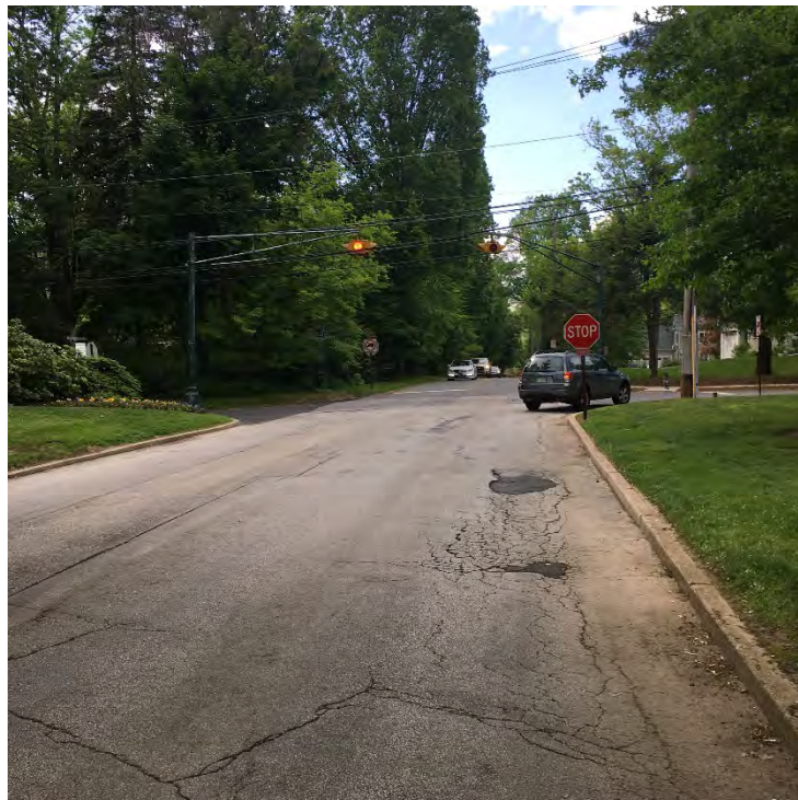
Photo # 2 - Description: Westbound Strafford Road
