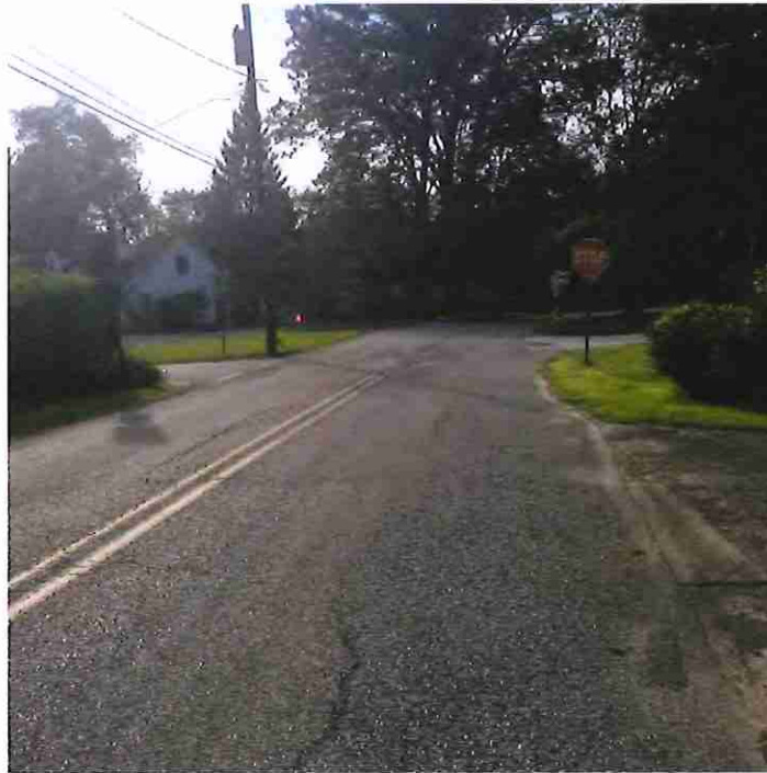
Photo # 1 - Description: Eastbound Strafford Road
