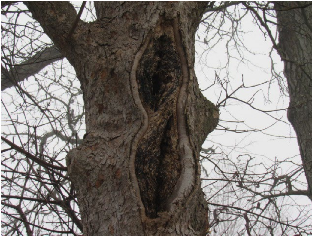
Photo 17, Sycamore Maple with stem decay. Removal recommended.
