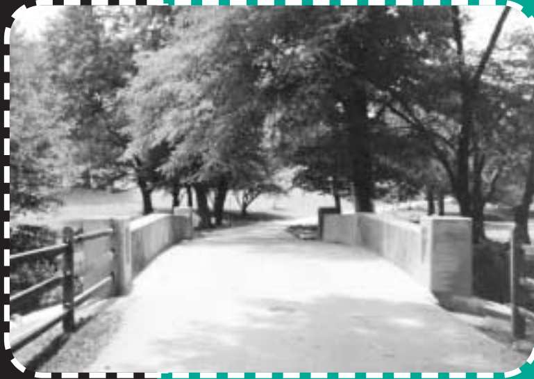
The bridges at the Willows were renovated, along with the pond and courtyard. Decorative tiles adorn the posts on the bridges.
