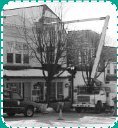
Public Works employees install new decorative streetlights on N. Wayne Avenue.
