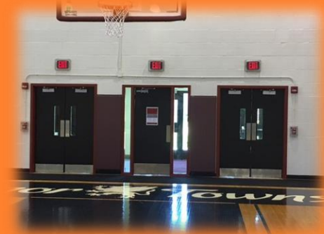
Interior Wall Padding & Painting - 2016
