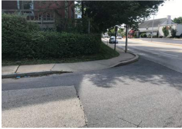
Photo 7: Westbound Roberts Road, looking left.
