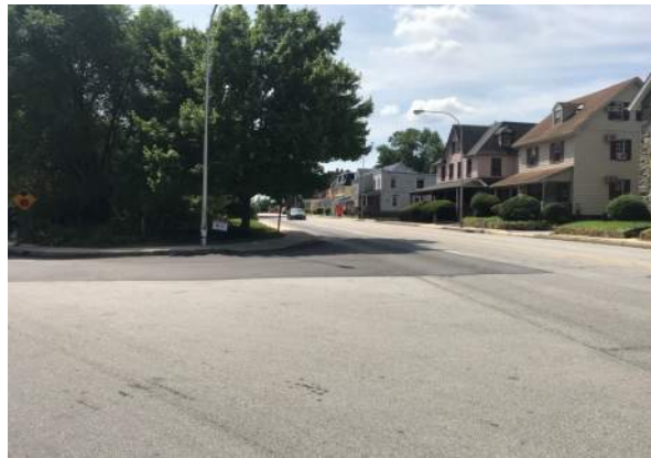
Photo 9: Westbound Old Lancaster Rd, looking left.
