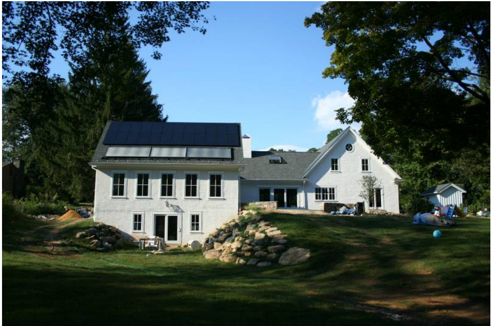
Back: South Façade w/ one of two 'out buildings'
